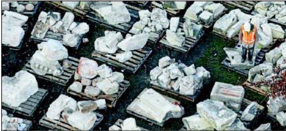
Neat piles: Rubble from the cathedral, above and left, is sorted and some stone will be saved and used for repair work.
