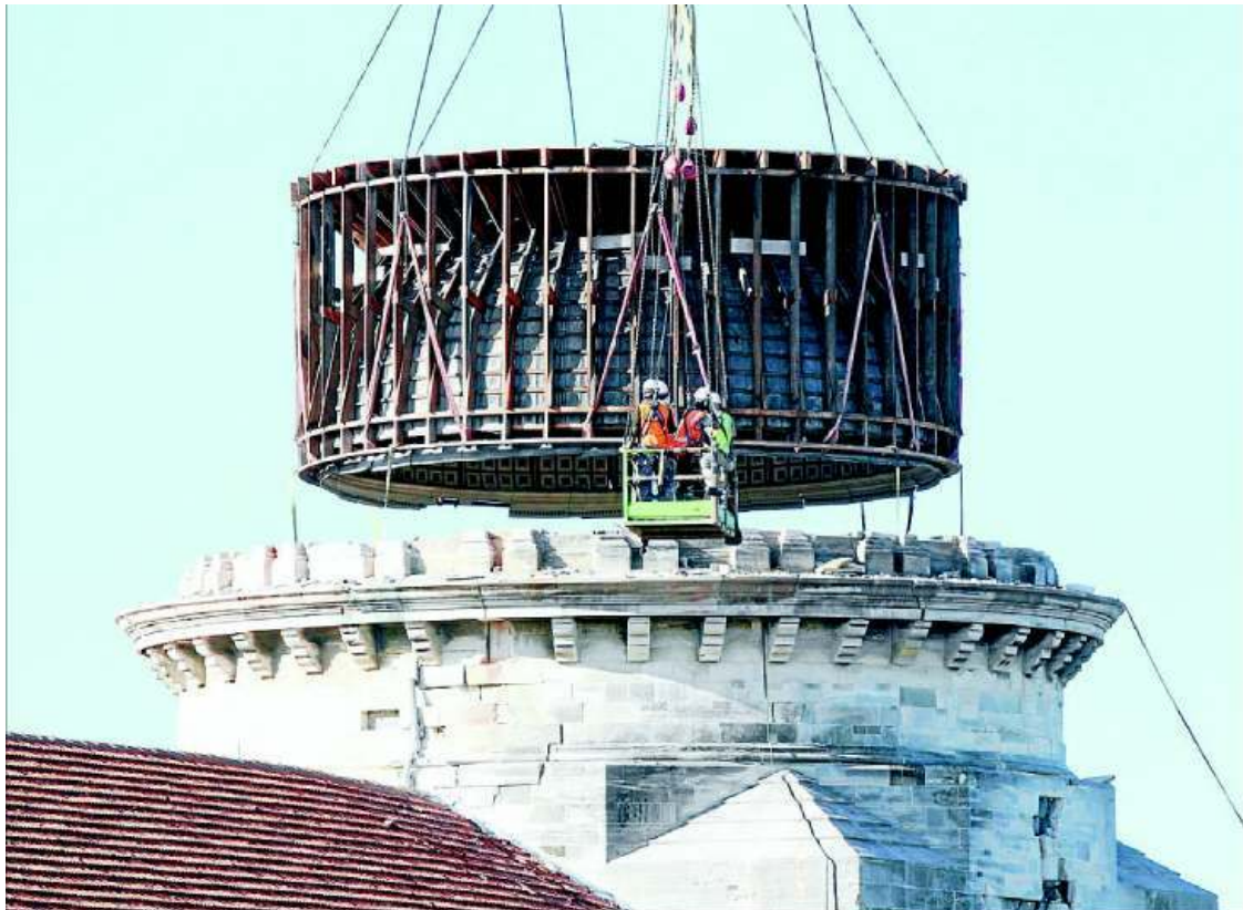
Undamaged: The copper dome is lifted out of the Cathedral of the Blessed Sacrament. Photo: STACY SQUIRES
